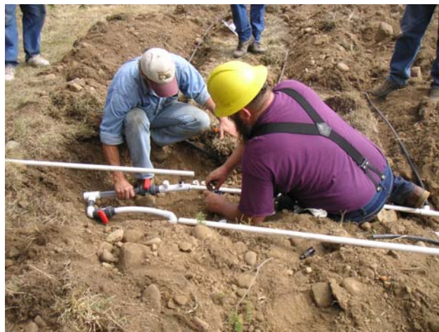
Laying Down the Line
