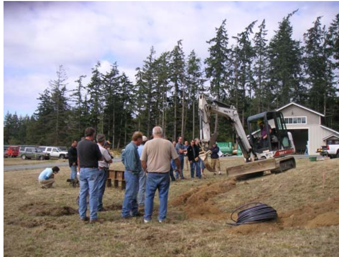
Finishing the Trenches
