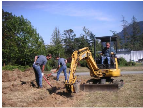
Backfilling in a Cloud of Dust
